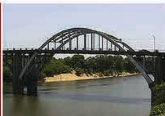
The Edmund Pettus Bridge, Selma, Alabama Photograph courtesy of the Alabama Historical Commission
